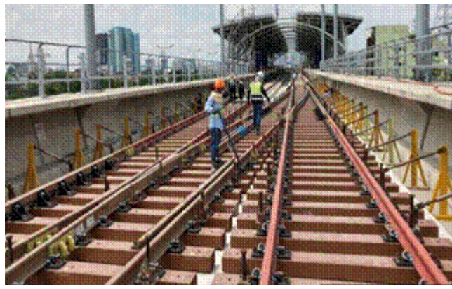
Turnouts on Concrete Bridge
