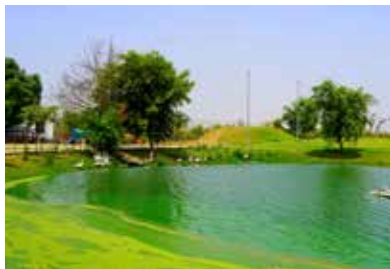
Rainwater harvesting center constructed by MCF
