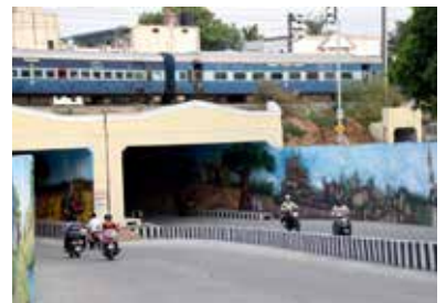
Road Over Bridge to enhance Safety
