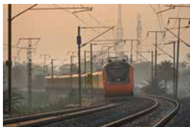
100% electrification works completed by South Eastern Railway
