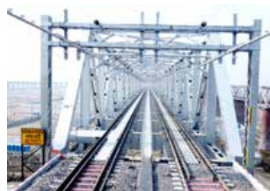
Newly constructed double line rail bridge over river Ganga in Prayagraj
