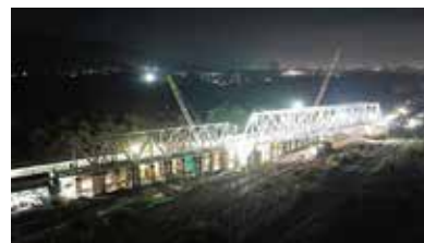
DFCCIL successfully launches open web steel Girder on its largest RFO
