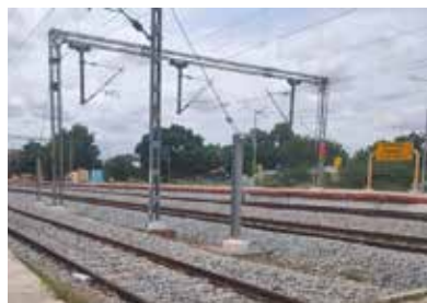
Railway doubling works, IR
