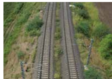
Railway doubling works
