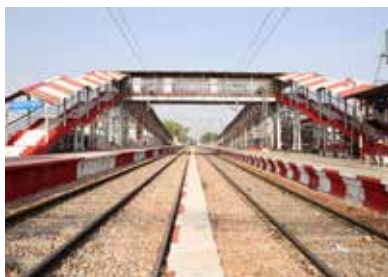
Foot over Bridge at Hathras City Railway Station
