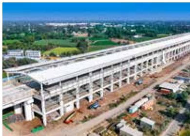
Under Construction Annad Bullet train Station in Gujarat.
