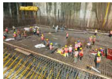
Under-construction Mumbai Bullet Train Station
