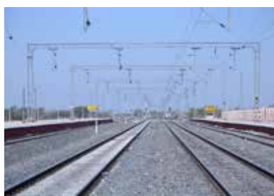
Accomplished 100% Electrification work of Broad Gauge Network, WR.
