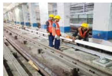
Replacement of Steel Third Rail by Aluminium Third Rail
