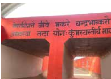
Road under Bridge at level crossing between Jhusi-Ramanathpur Stations.
