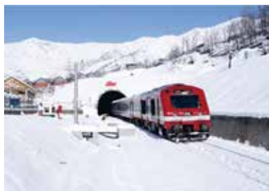
Pir Panjal Tunnel, Jammu & Kashmir
