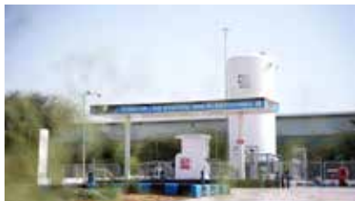
LNG Station, Kathuwas Railway Station.
