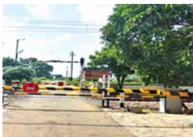
Electrical Operating Lifting Barrier with Sliding Boom
