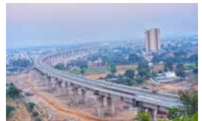
Dedicated Freight Corridor
