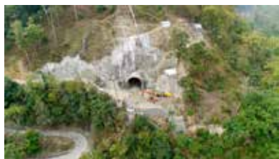
Tunnel work at Sivok Rangpo, IRCON
