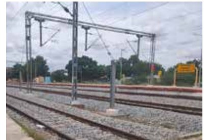
Railway electrification works
