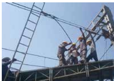
Electrification Work under the Mission Electrification
