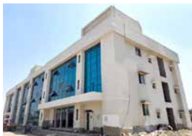
Combined Terminal Building of Muzaffarpur Station under ABSS
