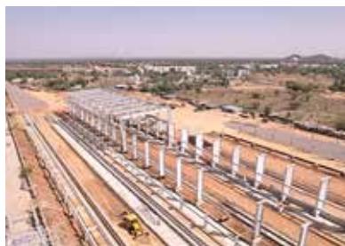
Construction of Coaching Terminal
